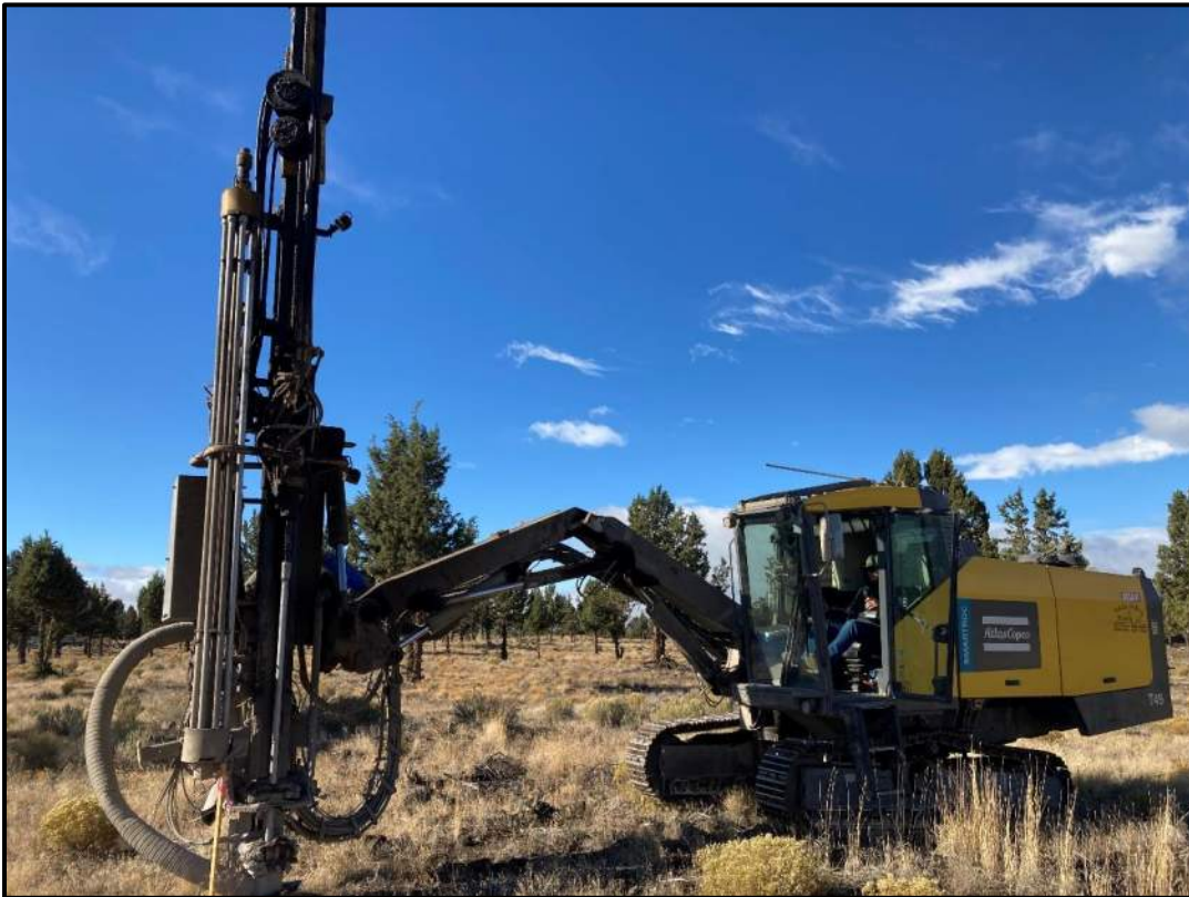
Air-track drilling performed with Atlas Copco T-45 drilling rig.
